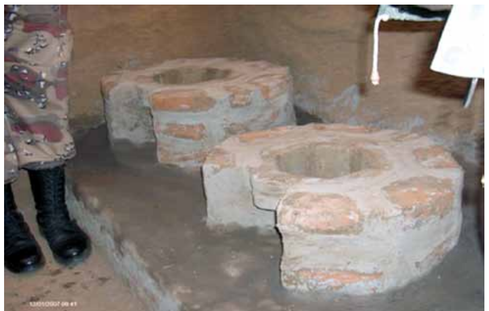
Energy-saving Jiko (Rondereza) constructed as part of Quick Impact Project in Kabkabiya, North Darfur, by Rwabatt 4 when the author was the Sector CIMIC Officer.
